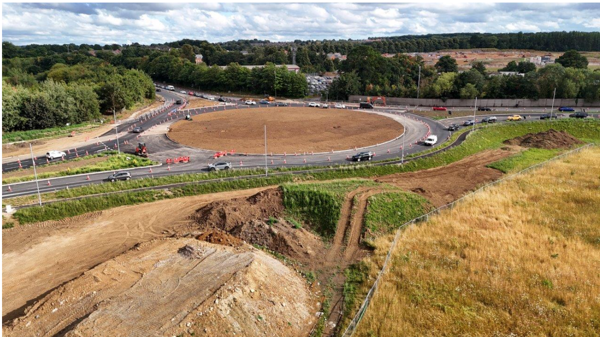
Looking southeast towards Coldharbour Roundabout
