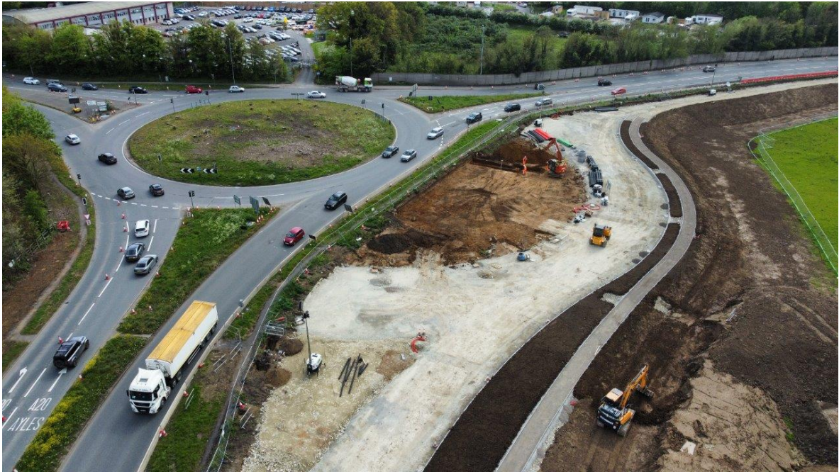
Looking south towards Coldharbour Roundabout
